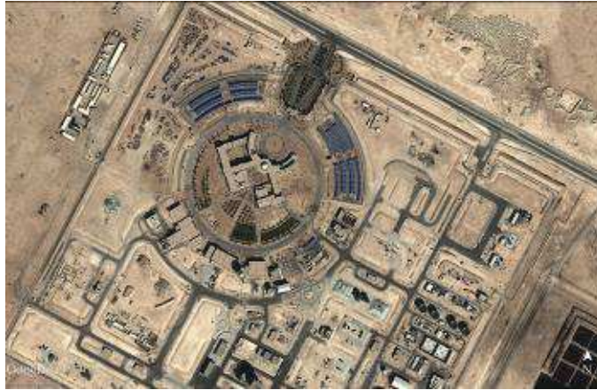
The Ras Laffan Emergency & Safety College project © Google Earth Imagery © 2013 Digital Globe. January 17, 2013. 25.883702, 51.431839
