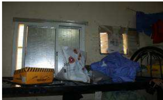
Hole in the wall where an air conditioner should be installed. Camp in Doha's Industrial Area, October 2012 © Amnesty International
