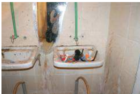
Workers' bathroom without functioning sinks. Doha's Industrial Area, October 2012 © Amnesty International
